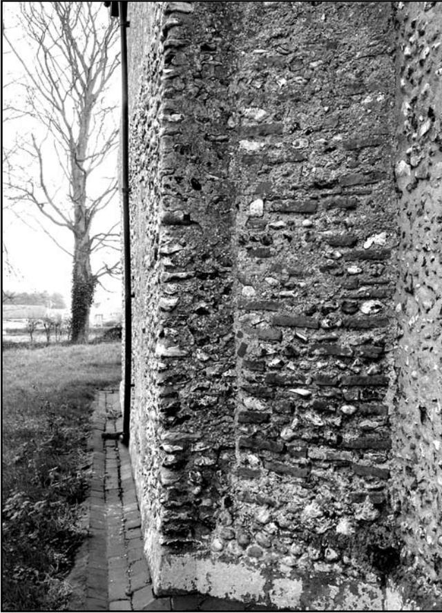
**Photograph 2. North-west corner of the nave where it abuts onto the tower, showing the flint quoins of the Saxon wall of the nave and the fillet of brick and flint bridging the corner between the nave and the tower.**
