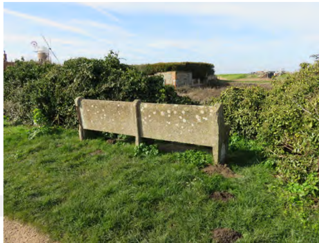
This reinforced concrete seat on the Coast Road is in poor condition and detracts from the quality of the area
