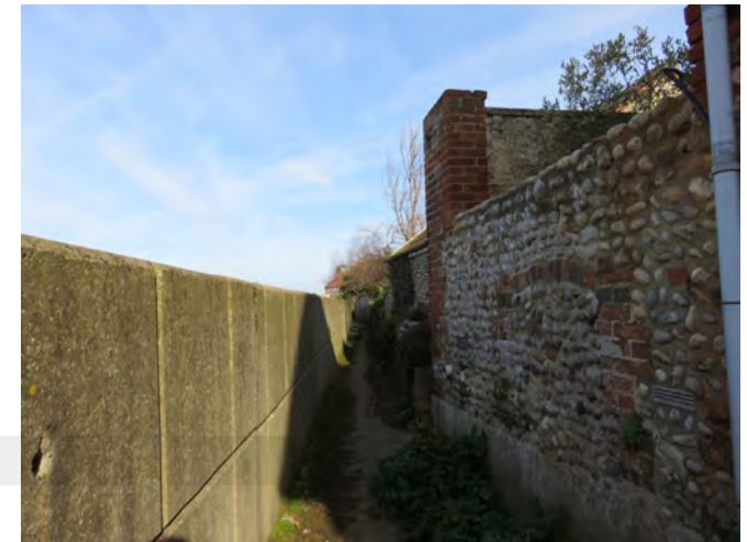
The concrete flood defences are not an attractive addition to the village but a very necessary one
