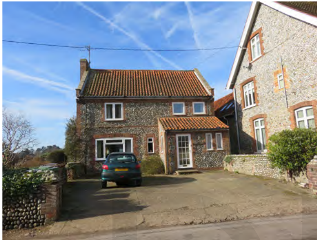
Front garden replaced with concrete. Not only does the concrete surface detract from the Conservation Area but also the loss of a boundary demarcation.
