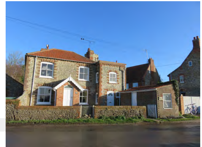
The boundary wall is in poor condition and spattered with mud. The gate should also be reinstated
