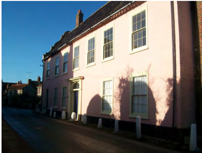
The Gables, High Street. A high-status house to a classical design.
