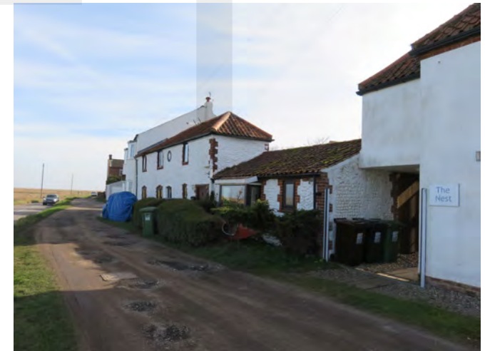
Potholed tracks detract from the setting of the buildings and are a potential source of injury for pedestrians
