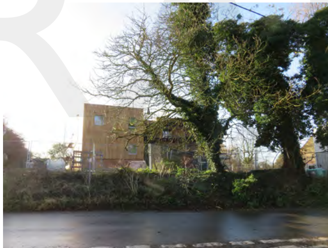
The scale and massing of this new dwelling are out of keeping with the other dwellings around Cley Green and significantly detracts from views around the Green as well as the setting of the church and nearby historic buildings
