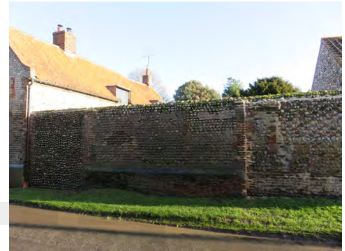
Grade II listed wall to Green Farm
