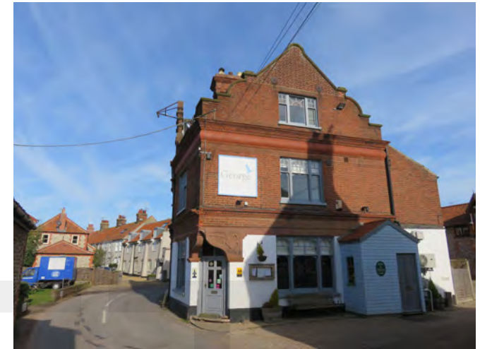
The combination of air conditioning unit, lights, alarm, junction box and signs create a cluttered appearance
