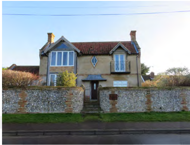
Detached modern house on Holt Road
