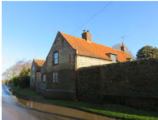
Green Farmhouse and boundary wall is soaked by passing cars driving through the water collected in a dip in the road
