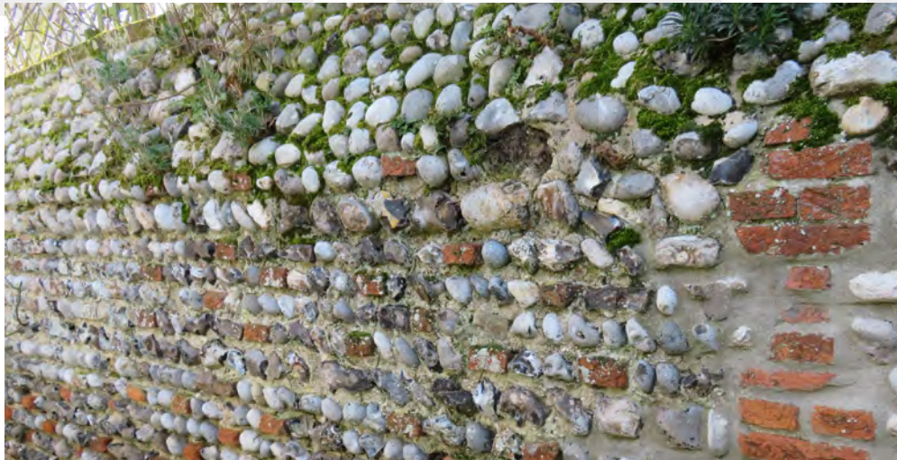
Flints will fall out of walls that are not well maintained. Vegetation growth causes damage to walls. Poor quality cement repairs affect the appearance of walls, especially where they cover the edges of the brick
