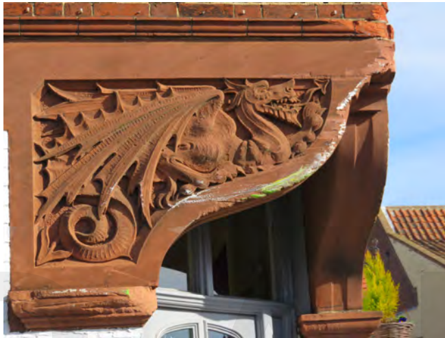
The terracotta dragon at the corner of The George shows evidence of damage from vehicles
