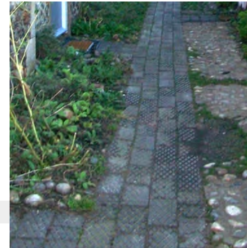
Detail of the paving to the footpaths
