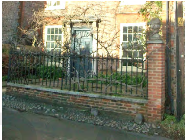
Listed wall and railings outside of Custom House
