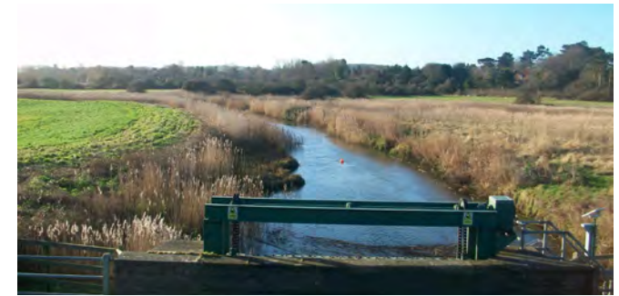
The River Glaven from the bridge on New Road, looking south
