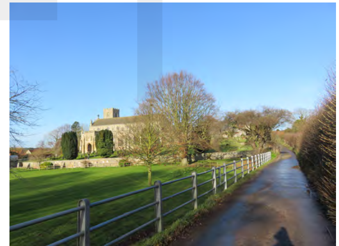
Railing to Church Lane
