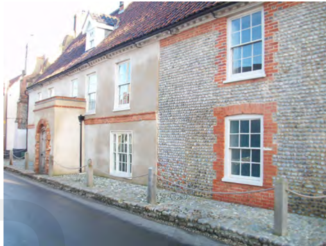
Wooden bollards protecting the façade of the house
