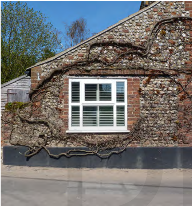
uPVC window on The Street. Its white colour contrasts starkly with the brick and flint work, while the top-hung casement is atypical of the Conservation Area
