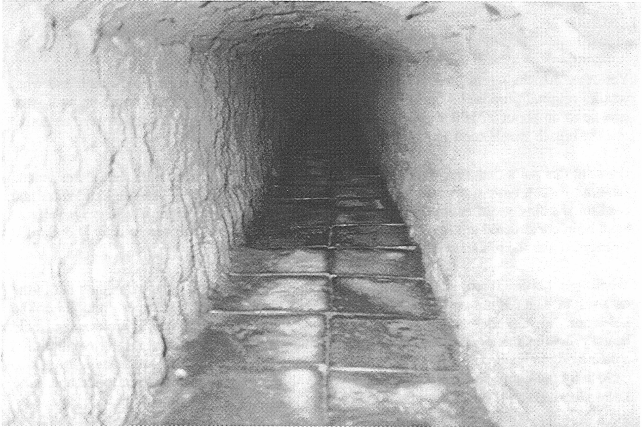
The tunnel - the view is the same in either direction
