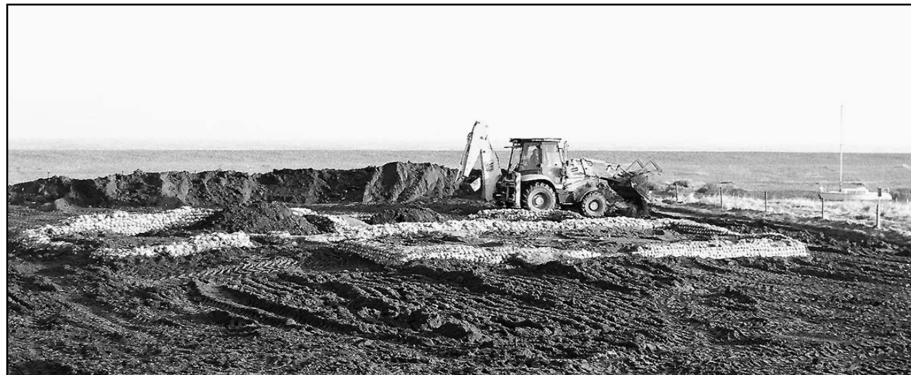
Photo 21. Excavation completed and the site backfilled. The next stage was cutting the new channel and filling in the cut so that in future access to the site will be from the shingle spit.
