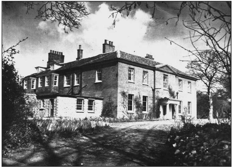
Cley Hall front elevation in c1960 showing the ‘sweet-room’ extension on the left.
