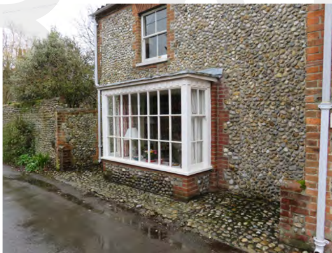
Cobbled floorscape on Chapel Lane is being damaged by vehicles
