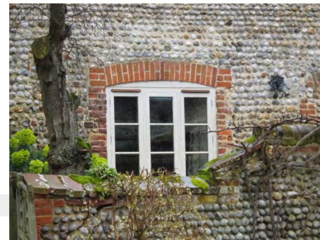
Window vents added to replacement windows detract from the appearance of the windows
