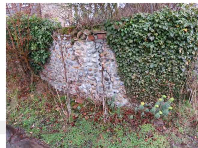
Damaged flint wall along The Street
