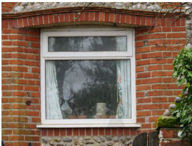
Example of an inappropriate uPVC window
