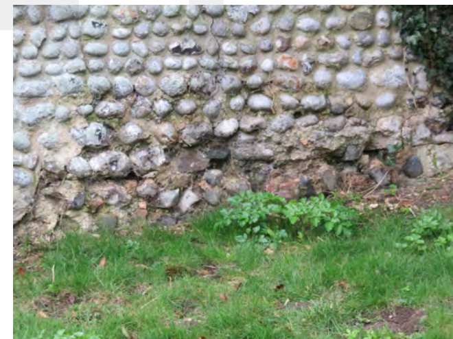
Failing flint wall on Leatherpool Lane
