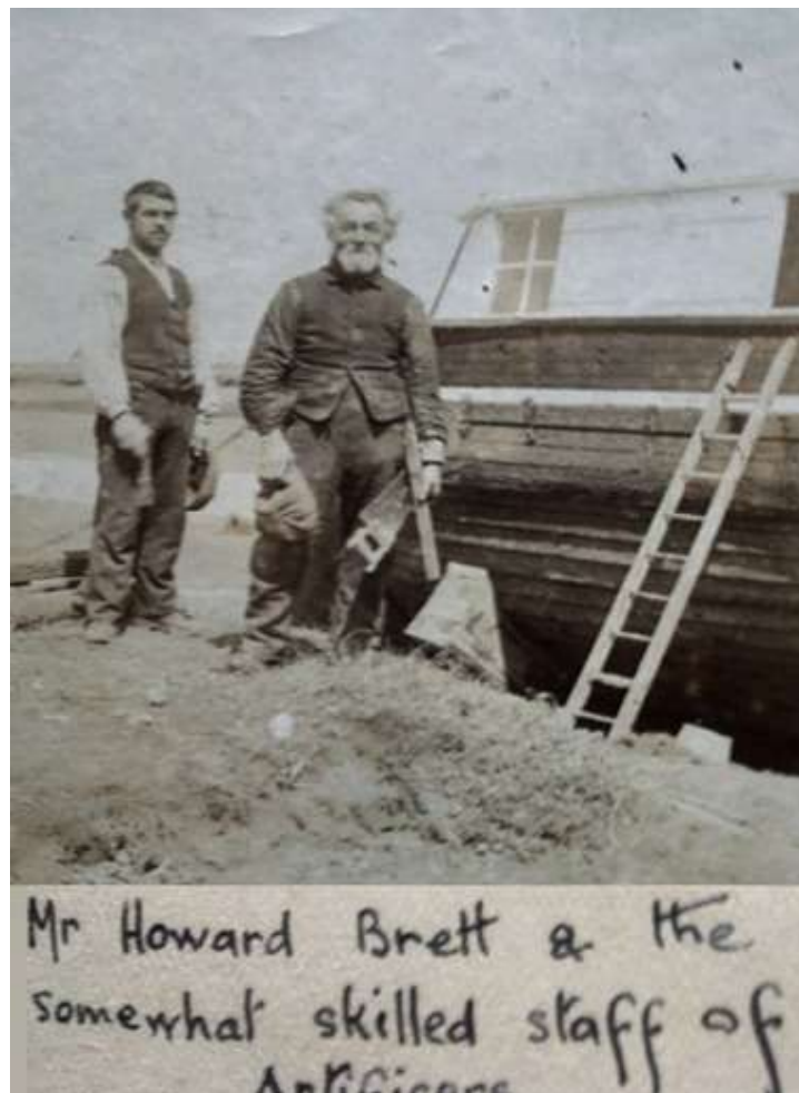
Howard Brett working on the conversion of the Gypsy Lass
