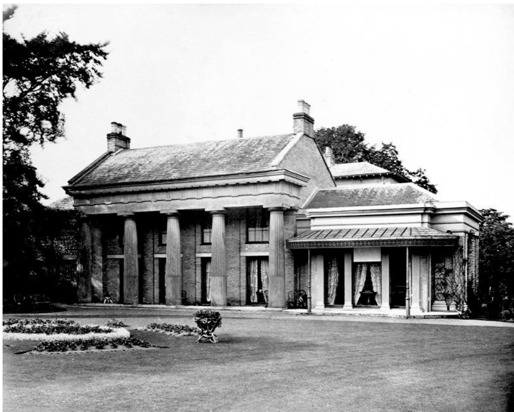
Letheringsett Hall's south front, showing the Greek Doric portico of 1809 designed by the local architect William Mindham. [photograph A.E. Coe of Norwich 1880]
