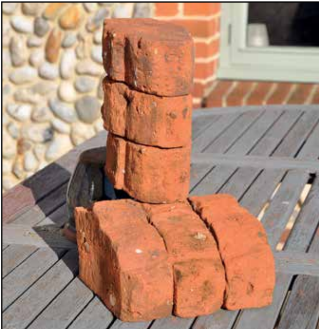
Photo of the brick mullion window frame at Barn Cottage. In re-using the wall the glass spaces had been blocked up with bricks.
