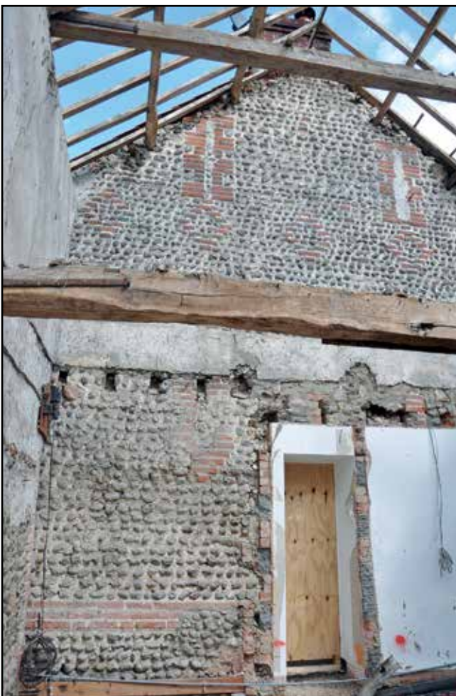
In putting the frontage in at Barn Cottage an old squared beam had been used, with mortice and tenon joinery. Glaven Farm is thought to have replaced a timber farm building. Nothing wasted, use what is lying about when heavy materials and poor road surfaces make transport difficult.
