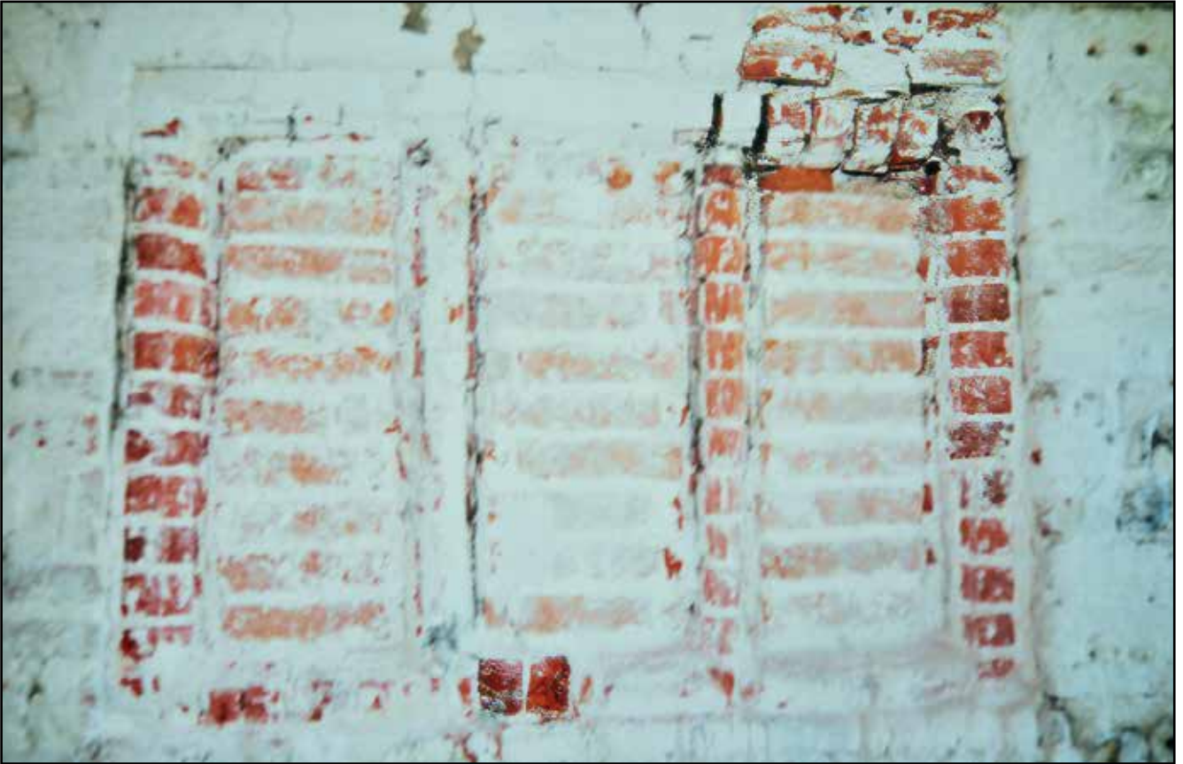
Photo of the brick mullion window frame at Barn Cottage. In re-using the wall the glass spaces had been blocked up with bricks.
