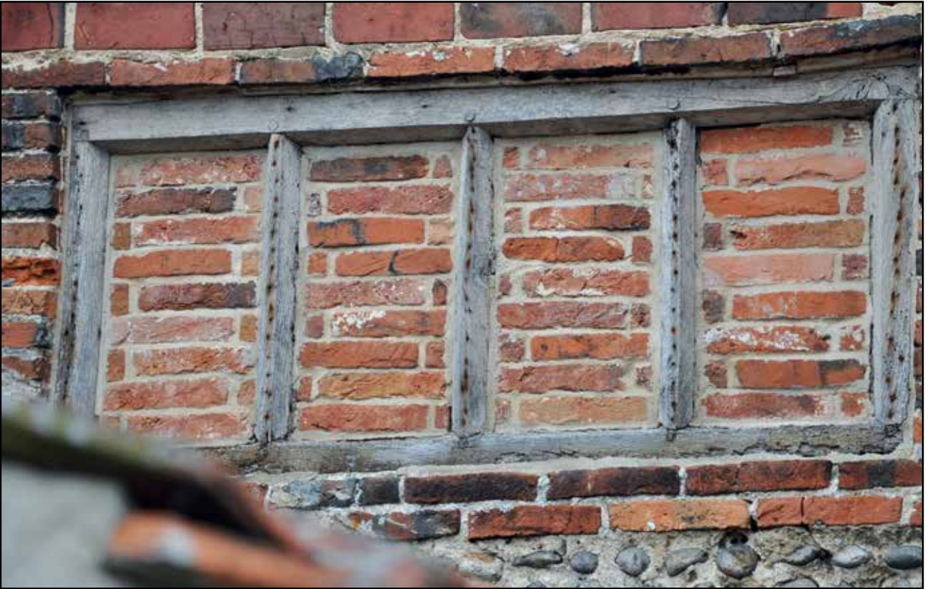
Bricked up oak-framed mullion window at Glaven farm. This, and another taken out completely, faced the river, as did the house itself until turned front to back, ca 1850. The mullion window had been covered by lath and plaster, after old bricks had been stuffed into the glass spaces. The blocking bricks were used at restoration to face off the spaces and display the oak frame.
