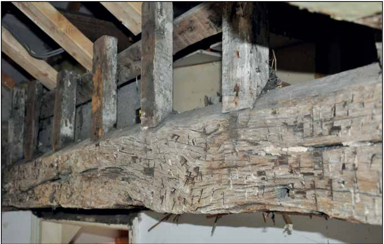
In putting the frontage in at Barn Cottage an old squared beam had been used, with mortice and tenon joinery. Glaven Farm is thought to have replaced a timber farm building. Nothing wasted, use what is lying about when heavy materials and poor road surfaces make transport difficult.
