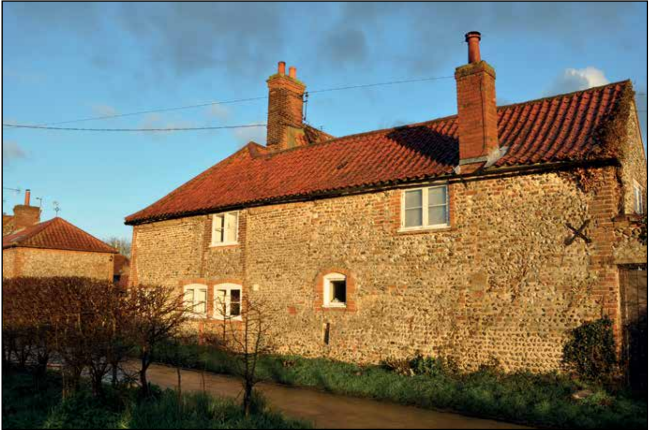
Glaven Farm along the lane, starting from part of a building at the south end, and progressing up the lane, and with a hip joint connected to the main building in a series of steps to form an L-shaped building. It's a puzzle to know the functions and uses of each addition along the lane.
